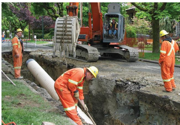
Figure 20: Excavation of Sewer Lines
